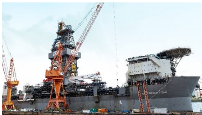
Photo: Construction of the 20,000 psi ultra-deepwater drillship continued in 2020.
