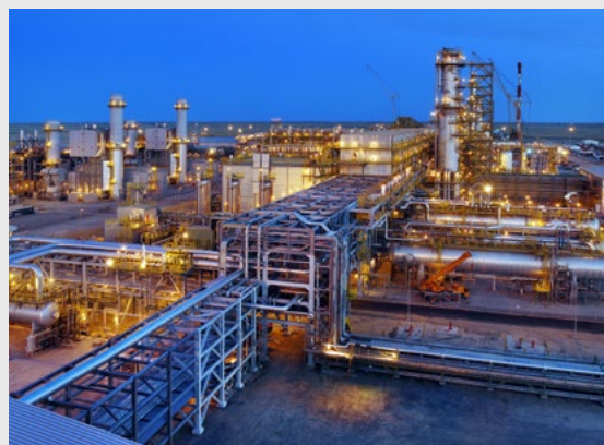
Photo: TCO utilizes data analytics and automated performance monitoring to improve returns.
