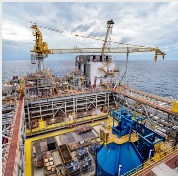
Photo: Efforts to enhance recovery at the Jack/St. Malo field include long distance tieback technology advancements.
